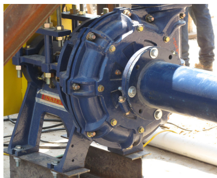
Warman® WGR™ slurry pump installation
