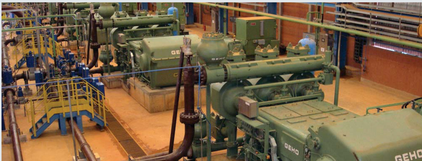
Figure 4. GEHO® positive displacement pumps used in a 245km long bauxite pipeline in parallel operation.
