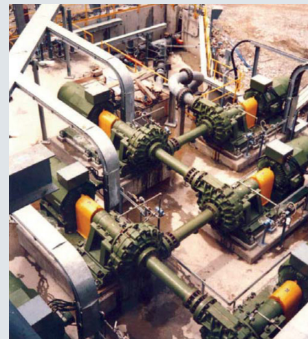
Figure 1. 8 stages of Warman®10/8 T-AHPP pumps on tailings disposal direct coupled at 740 r/min.
