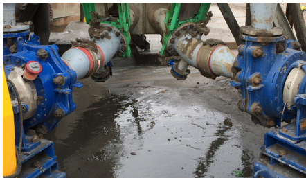
Top: Warman® WBH® 100 pump delivered on site
